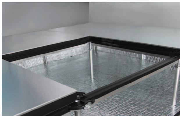
Condensation control is not only important within the plenum itself, but also for the surface of the adjoining under floor material. Insulation of the plenum provides protection against condensation on the lower floor ceilings.
